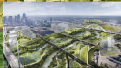
Trinity River Corridor Project - $2.5 B
