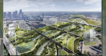
Trinity River Corridor Project - $2.5 B
