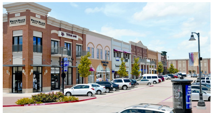
Arlington Highlands NEC I-20 & Matlock, Arlington, TX | 750,000 SF
